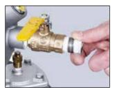
1. Install the ½" pipe nipple into the inlet of the ball valve. Use Teflon tape or thread sealant on the threads on both ends of the pipe nipple.
