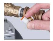
3. Install the ¼" push-to-connect elbow into the ¼" outlet of the tee. Use Teflon tape or thread sealant on the threads of the elbow.
